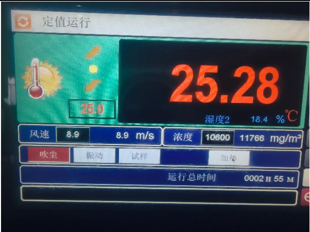
No.6-9 Control panel
